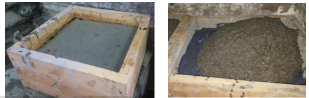
Figure (2) Fabrication of sample substrate concrete and repair concrete
